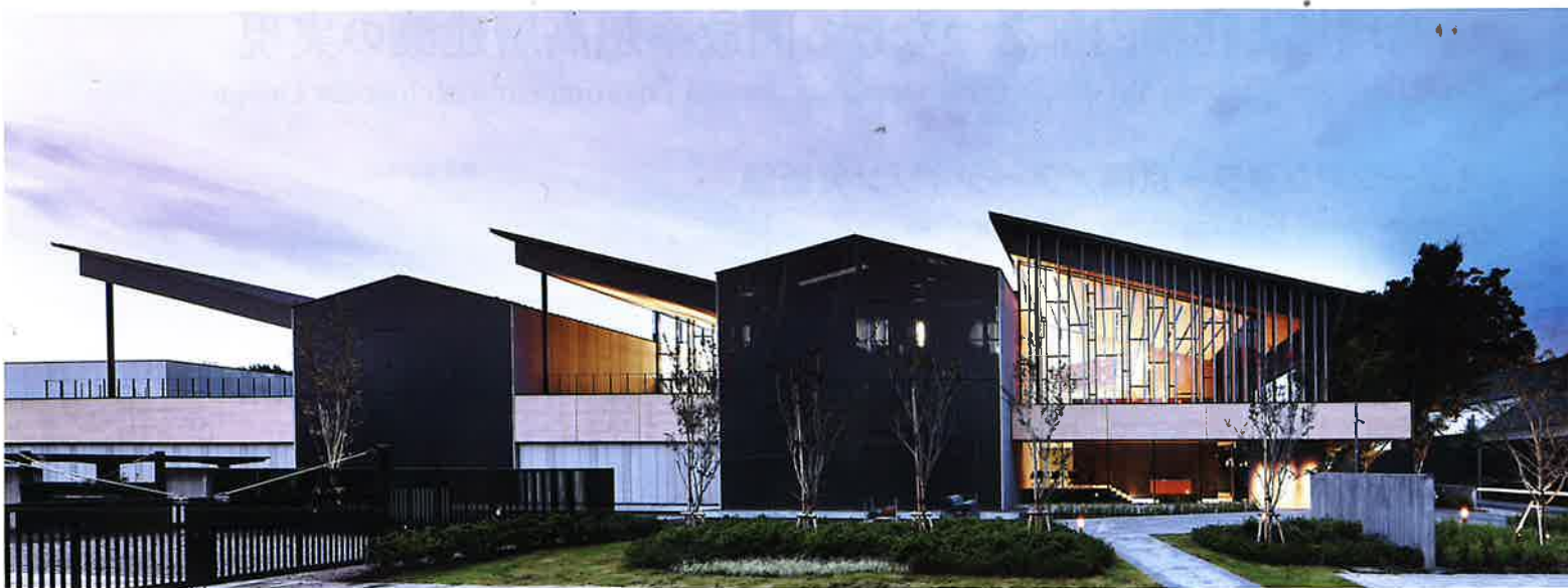
屋根は切妻屋根の集合体をベースとし、市松状の吹き抜けに合わせて屋根をめぐりあげ、光と風を立体的に取り入れている Roof design is a compilation of gable roofs, with elements that pivot to align with a checkered pattern of voids, thus sculpting the entry of light and wind into the building in a three-dimensional manner
